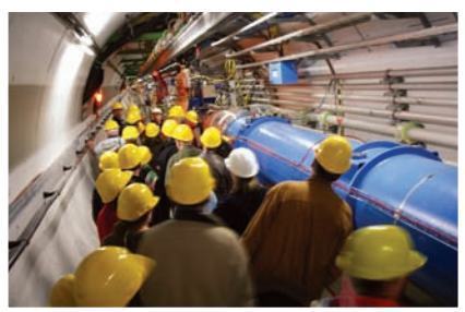
The LHC tunnel.
