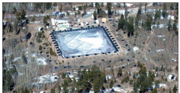
Fig. 1b. Aerial view of the Milagro gamma-ray observatory. The central reservoir is surrounded by 175 water tanks. (Courtesy Ulisse Bravar.)
